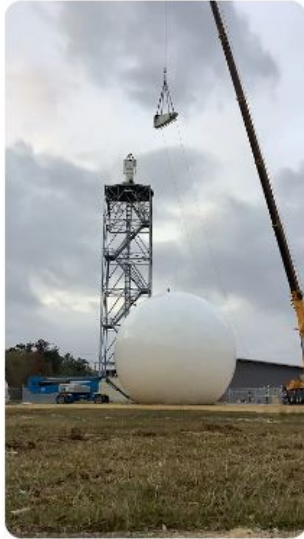
Lifting the radome onto the relocated KHDC radar... 639 views
