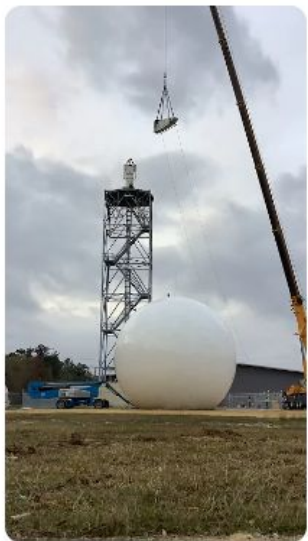
Lifting the radome onto the relocated KHDC radar...
