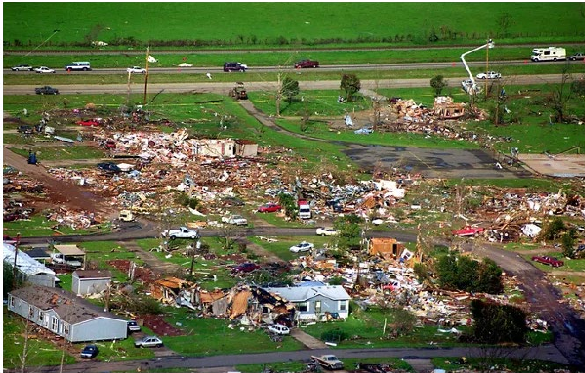
Rubble and debris is all that is left of the Hay Meadow Mobile Home Estates in Bossier Parish, La. after a tornado hit north Louisiana April 4, 1999. The Times
